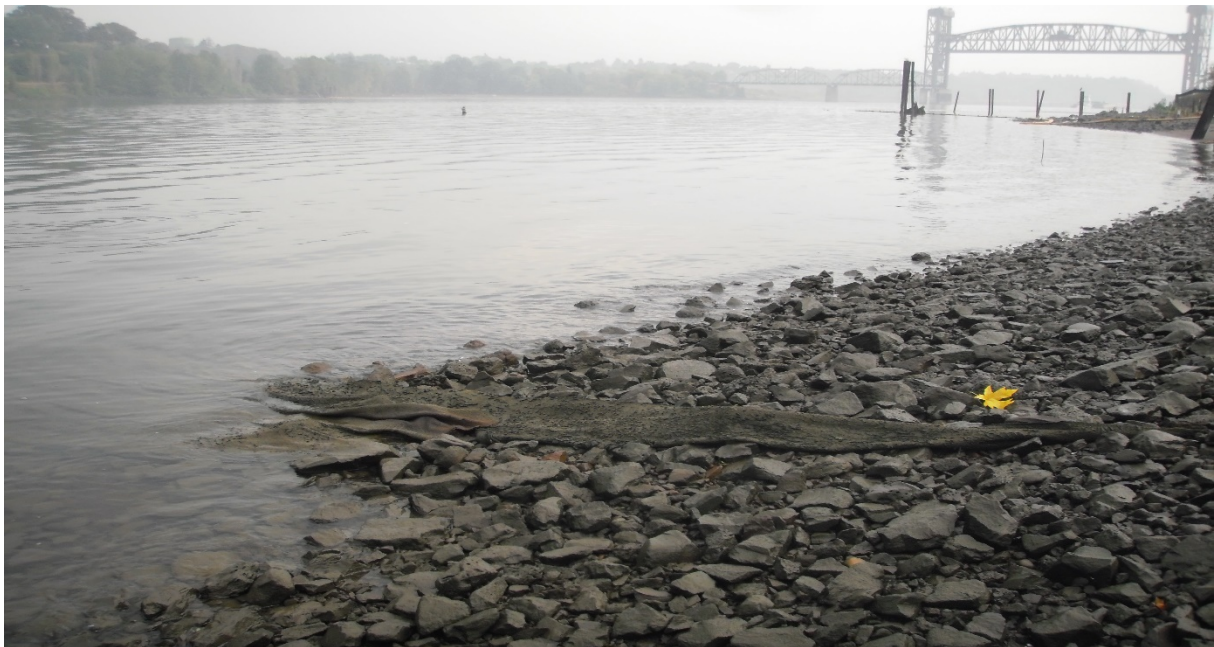
Photo 2 Exposed Organoclay Mat Material at the Upriver End of the Cap (9/18/2020)
