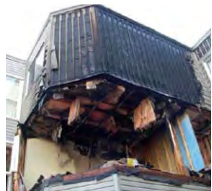
Smart meters will decrease illegal electricity diversion (shown here), keeping neighbourhoods safe from fires like the one that destroyed this house.
