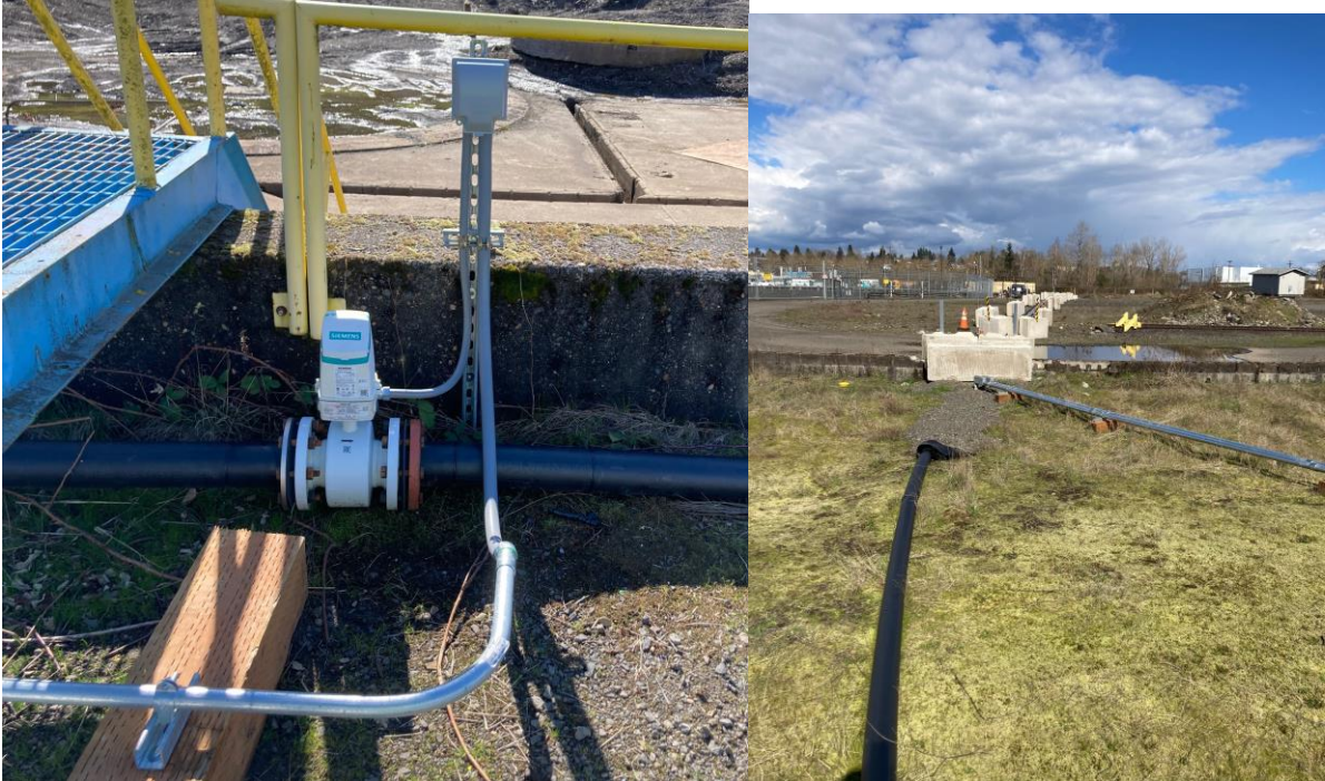
Flow Meter and Pipeline from Basin to Equalization Tanks
