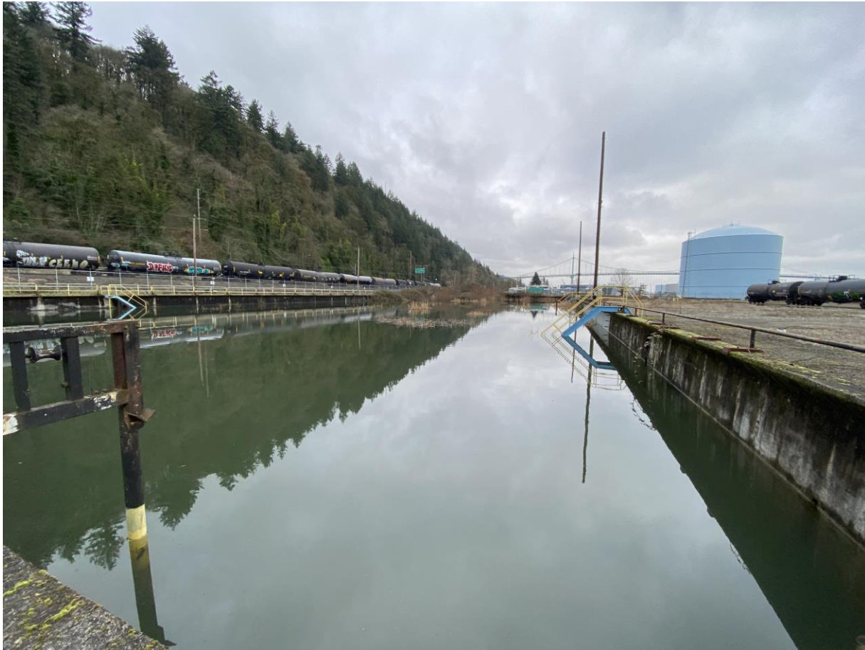
Figure 1: Former Koppers Basin Condition-January 21, 2021 Looking North
