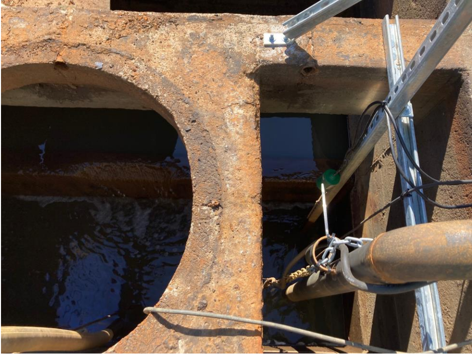
View of Pump in Wet Well (Green HIGH HIGH-LEVEL float shown)
