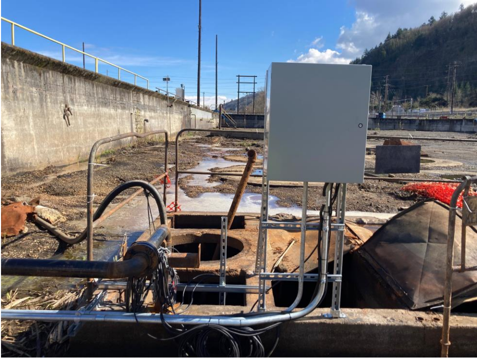
View of Pump in Wet Well (Green HIGH HIGH-LEVEL float shown)
