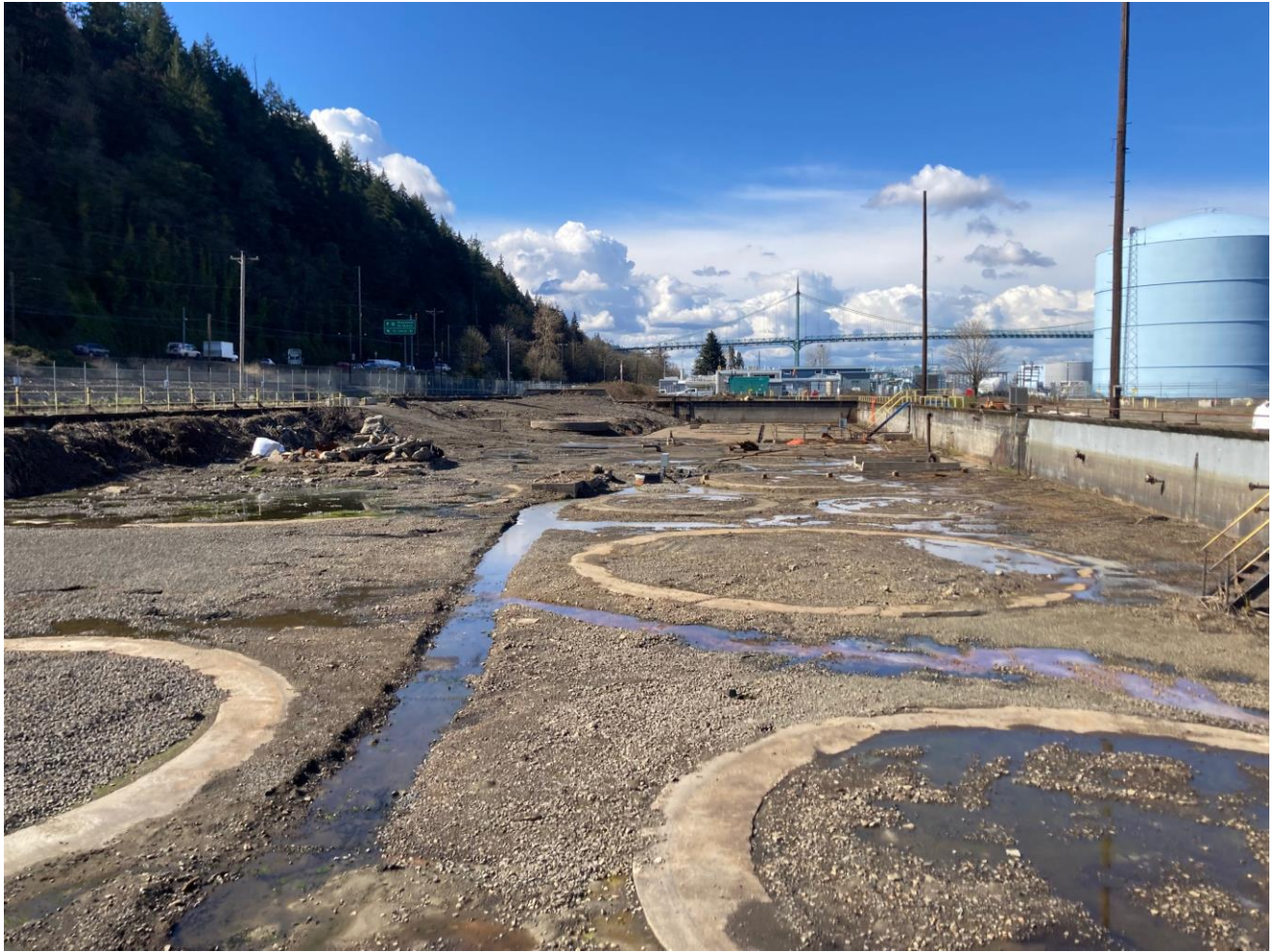
Figure 2: Former Koppers Basin--March 29, 2023, After Recent Rain Looking North
