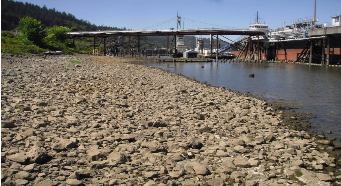
Photo 3 Conditions Immediately Downriver of Cap Area (8/17/2020)
