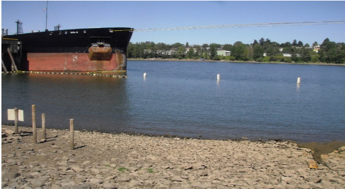
Photo 1 PacTerm Oil Boom Placement Around the Barge with Three Mariner Warning Buoys at Pilot Cap Area (8/17/2020)
