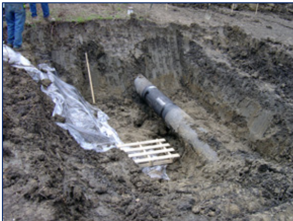
Fig. 3 Muddy trench with pallet for safe footing
