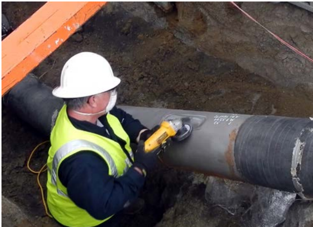
Fig. 7 ABIS personnel performing final polishing with handheld grinder/polisher
