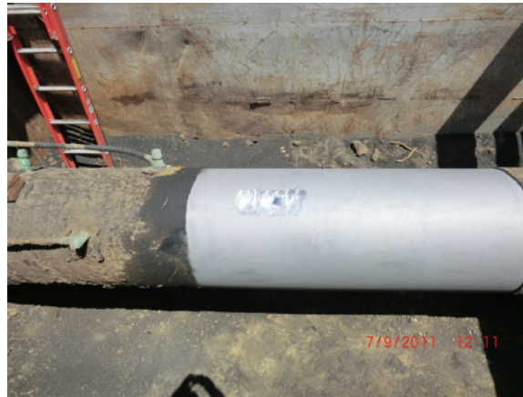
Fig. 6 Pipe after sand blasting
