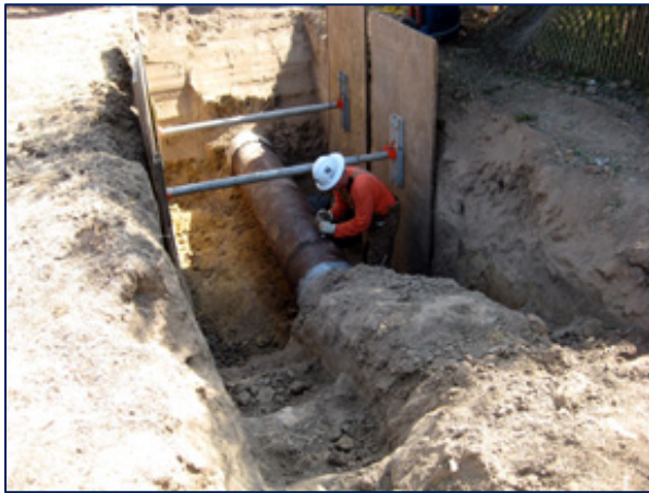
Fig.1 Reinforced trench with cut steps
