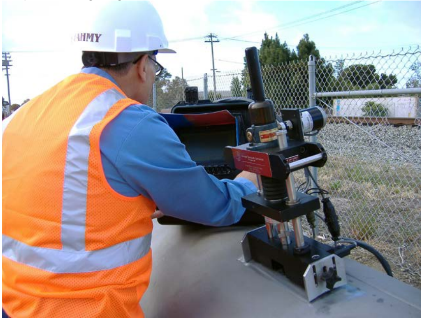
Fig. 9 Pipeline testing in the 12 o'clock position
