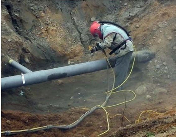
Fig. 5 Sand blasting pipe
