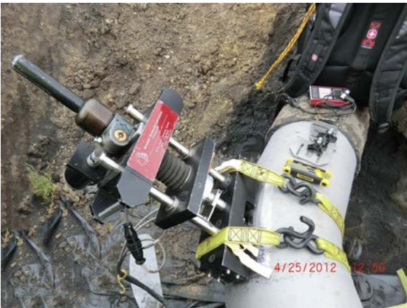
Fig. 10 Testing pipeline elbow (curved surface)
