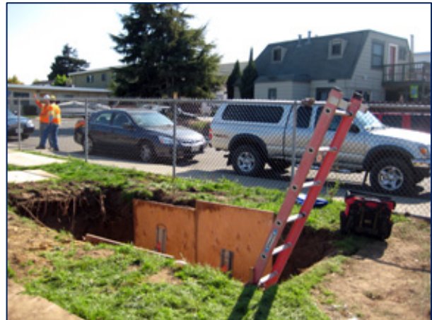
Fig. 2 Reinforced trench with ladder
