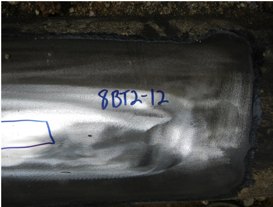
Fig. 23 Photos from Location 8BT2-12
