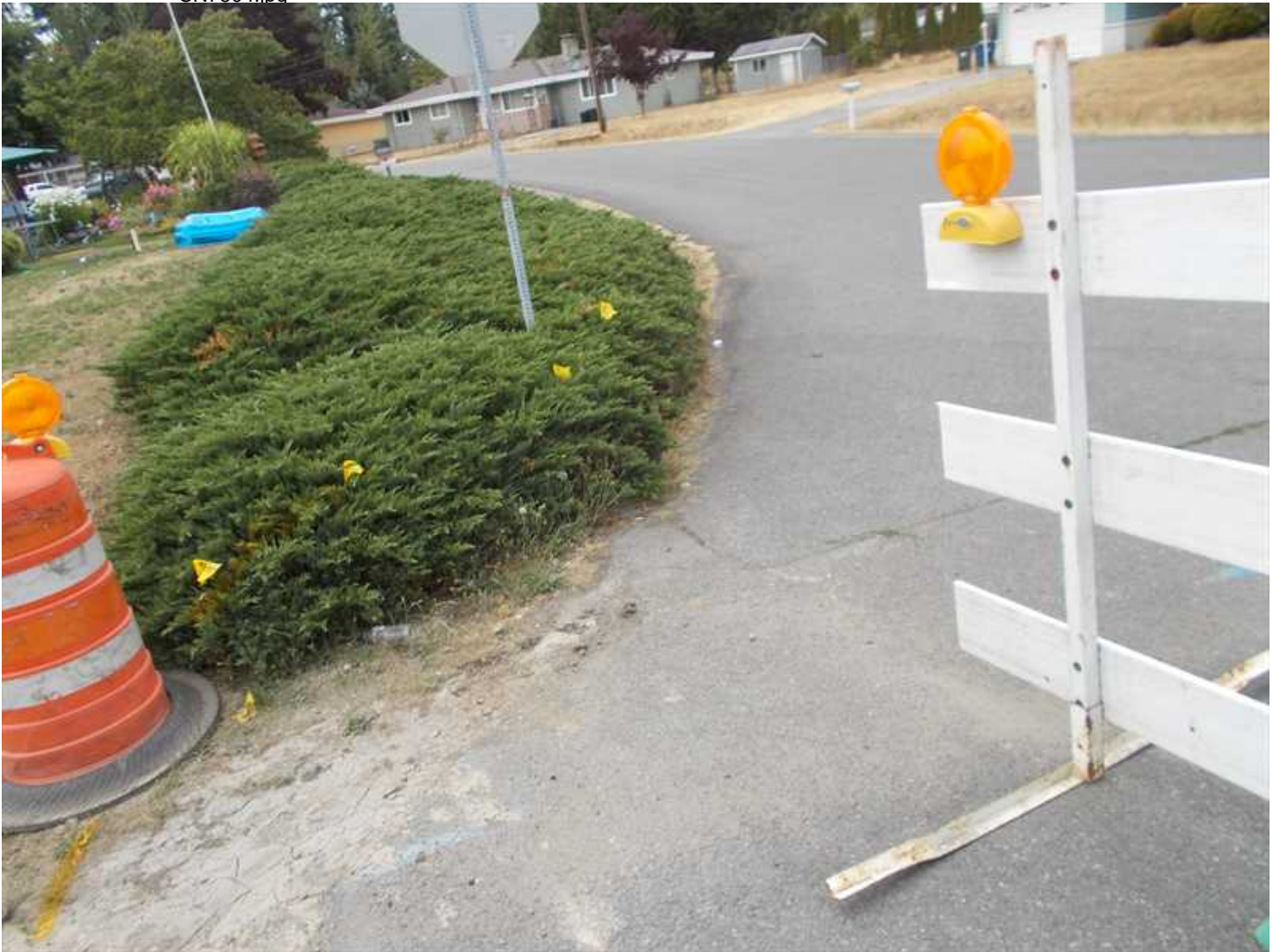
Property of United States Infrastructure Corporation Photo taken on 7/24/2015 3:35:30 PM
