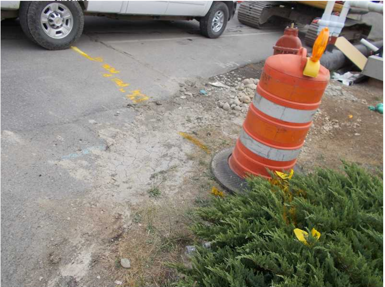
Property of United States Infrastructure Corporation Photo taken on 7/24/2015 3:35:22 PM
