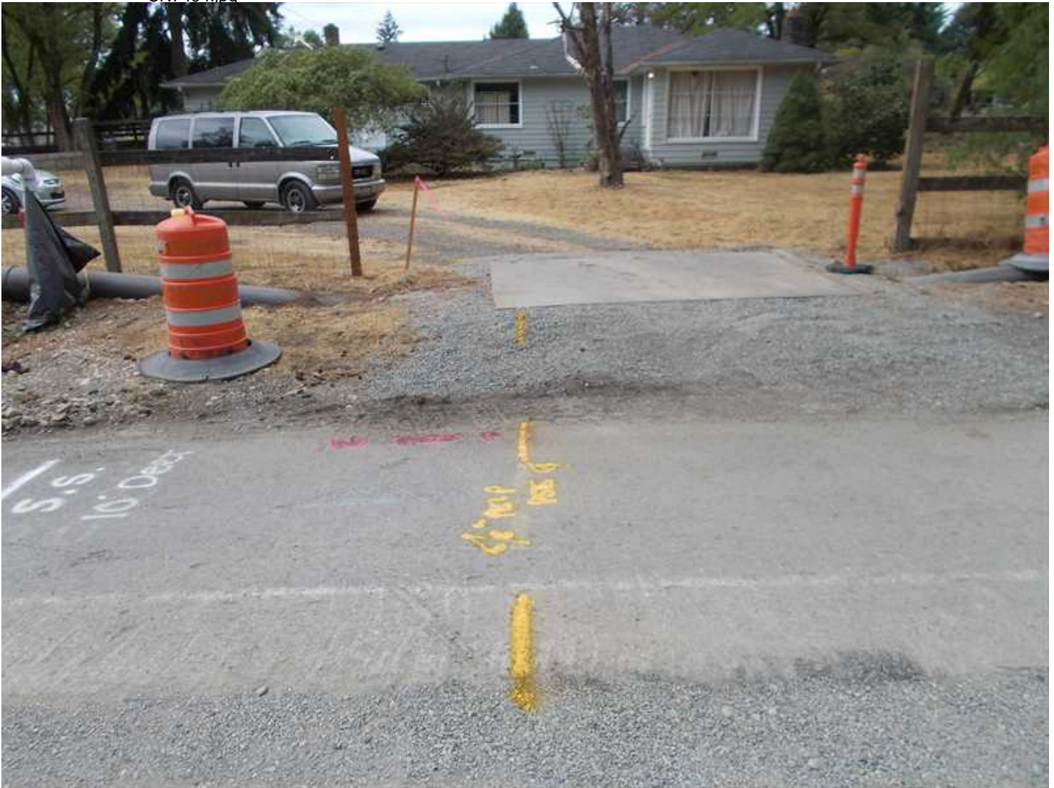
Property of United States Infrastructure Corporation Photo taken on 7/24/2015 3:28:06 PM
