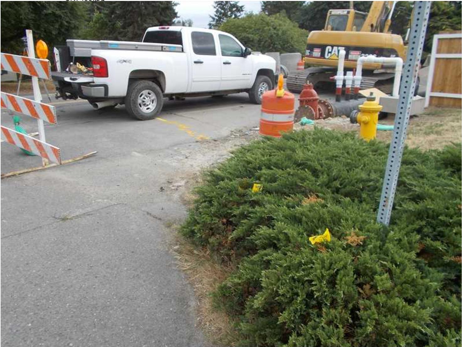
Property of United States Infrastructure Corporation Photo taken on 7/24/2015 3:35:16 PM
