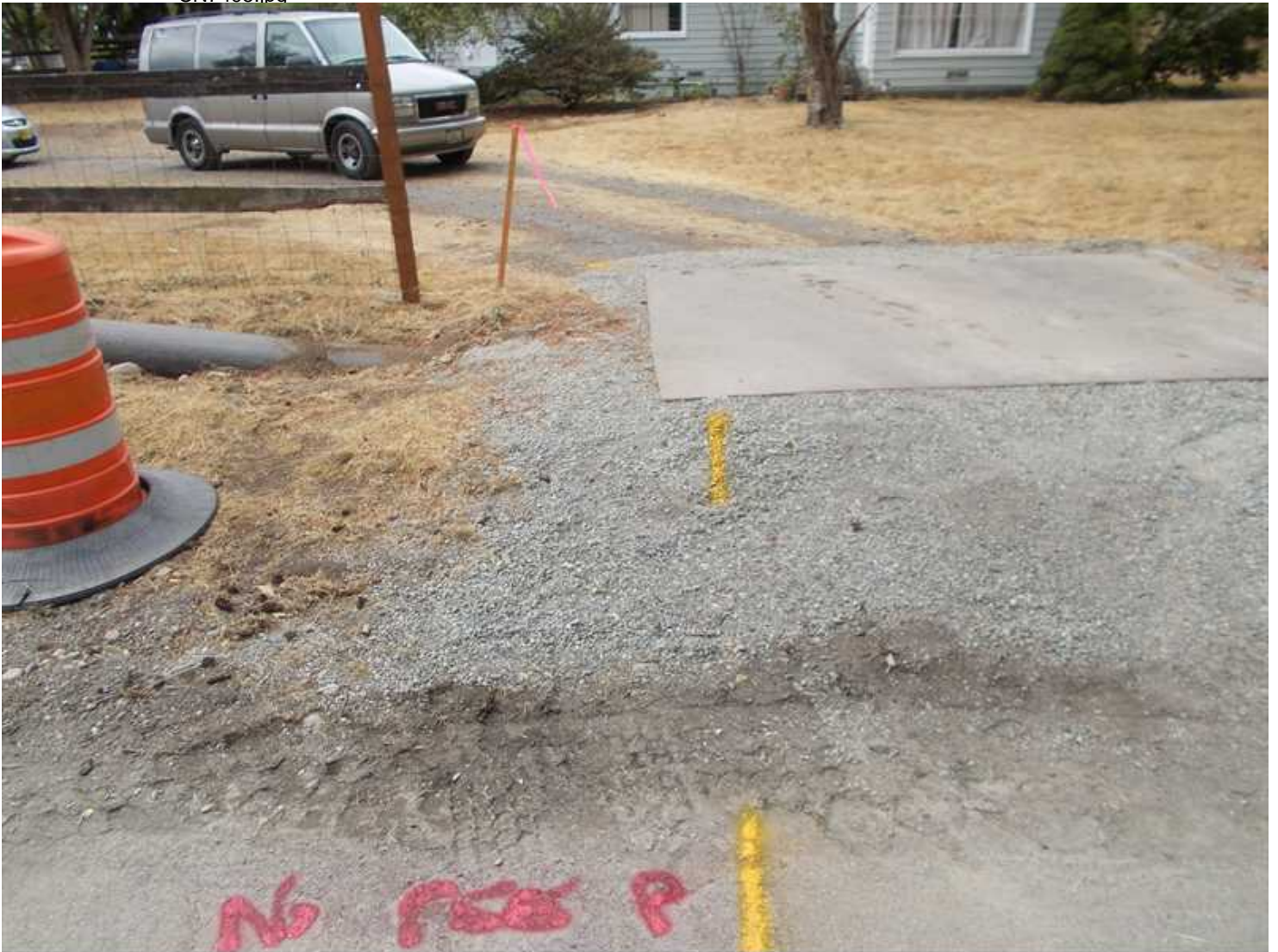
Property of United States Infrastructure Corporation Photo taken on 7/24/2015 3:28:08 PM
