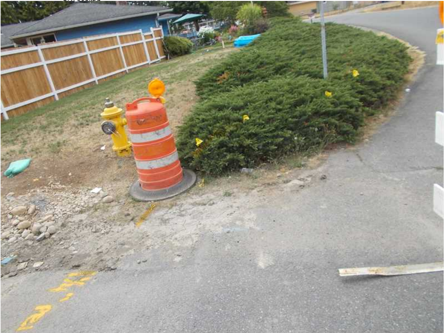
Property of United States Infrastructure Corporation Photo taken on 7/24/2015 3:35:28 PM
