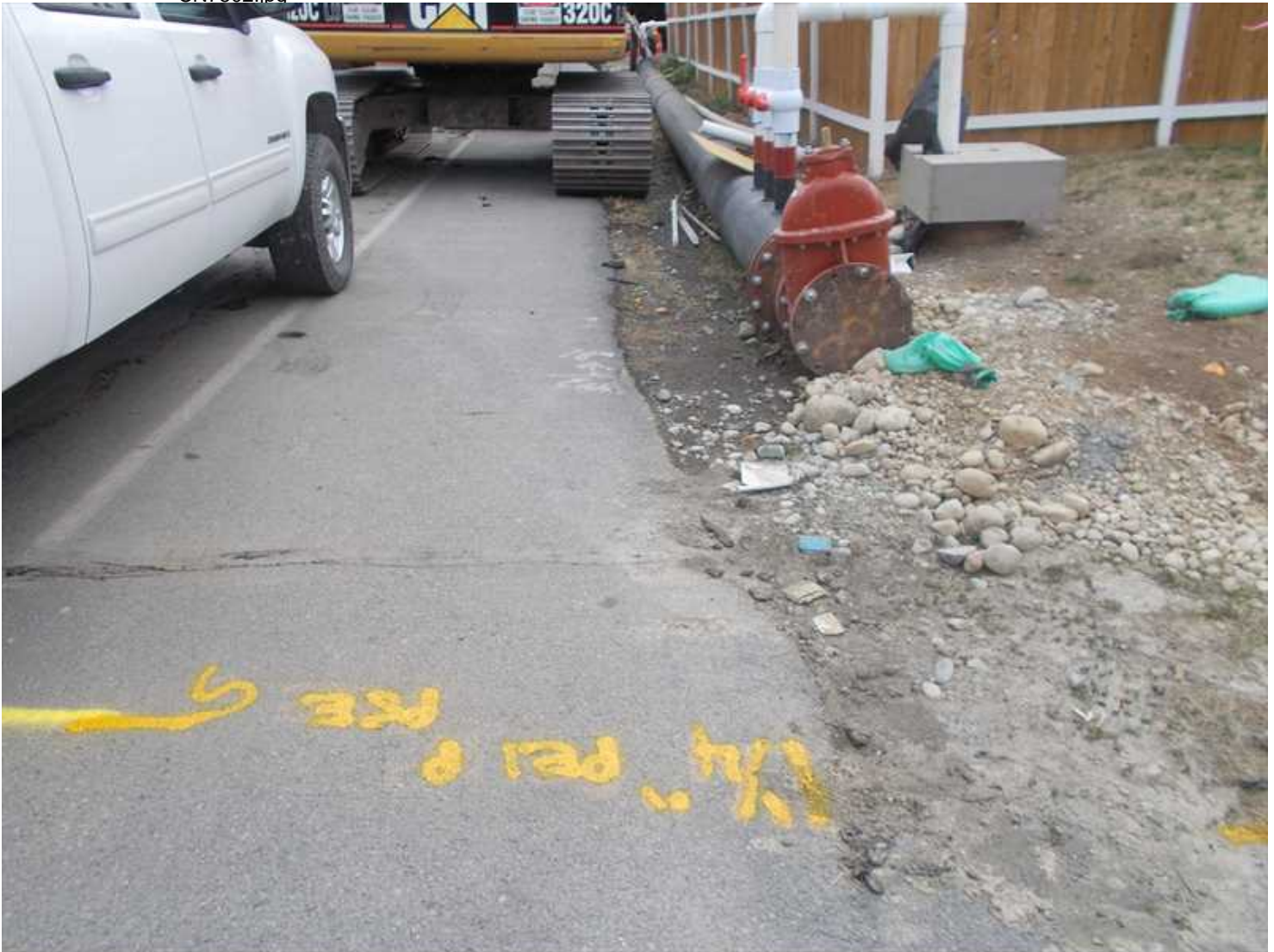
Property of United States Infrastructure Corporation Photo taken on 7/24/2015 3:35:24 PM
