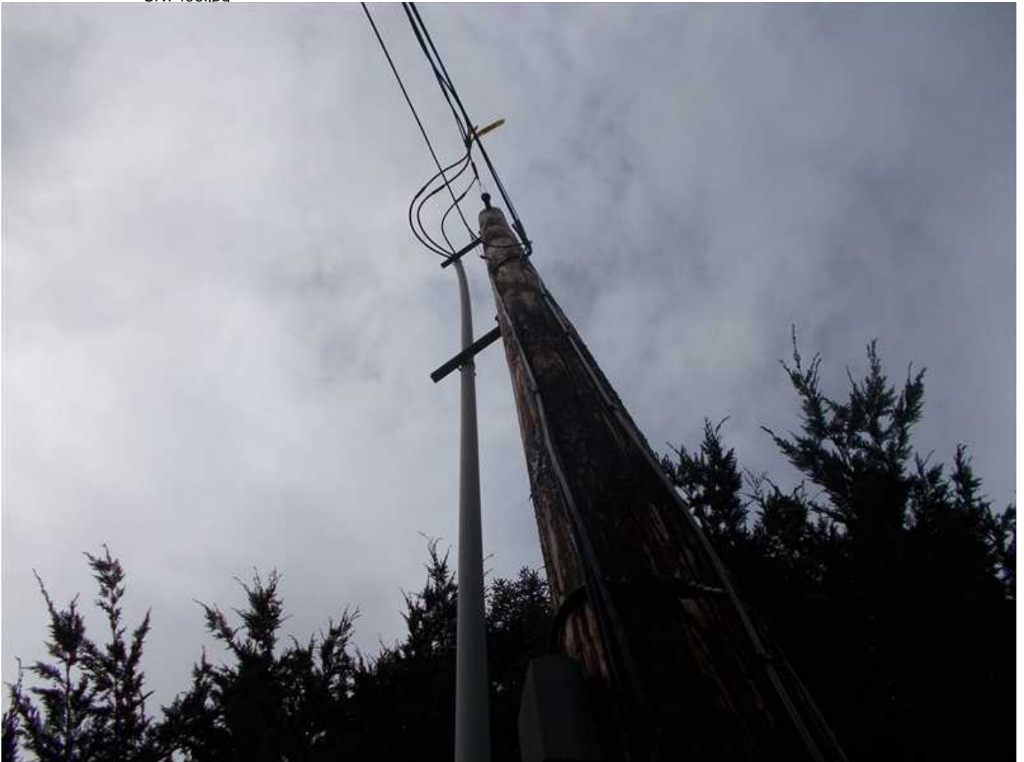
Property of United States Infrastructure Corporation Photo taken on 7/24/2015 3:30:48 PM
