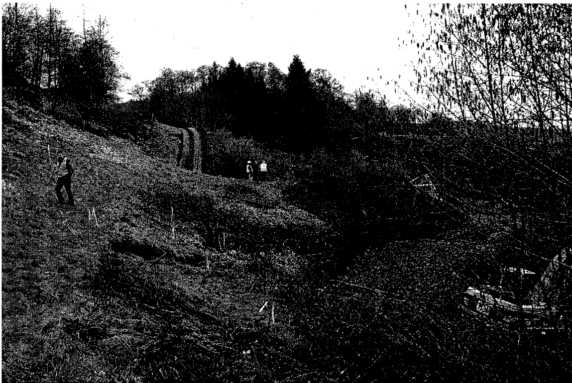
The K-B Pipeline is located below where the man in orange vest was standing on the left side of the picture.
