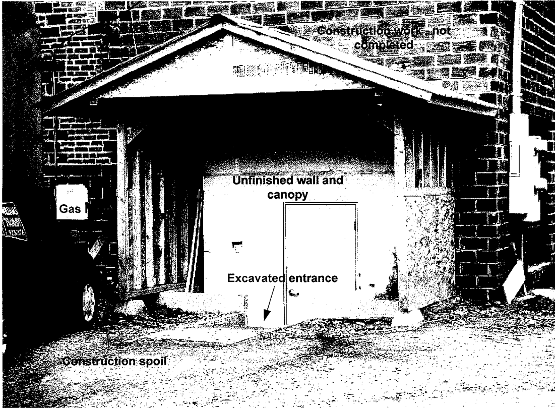
Rear of 600 N. Main Street showing building addition (Above)
